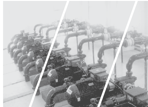
Boosting and Distribution of surface water
