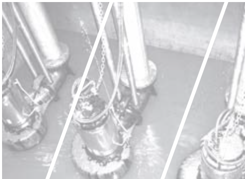
Wastewater Transport and Treatment
